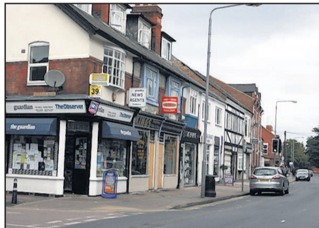
Chilwell Road shopkeepers will find tram construction work just feet from the entrances to their shops.
